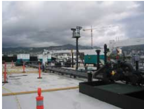
10T telescopic crane, 65 feet long, on oil barge
